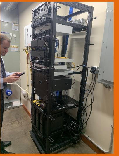
Engineering, technology, computer analysis, circuitry development and problem solving design can all be seen in this tower of power seen here. This is a project with one of his clients where they collaborated to develop and design a fully automated network with remote accessibility, backup power and multiple internet options.
